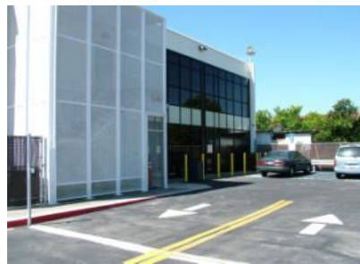
North elevation with new storefront
